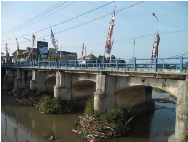
Picture 9. Condition of bridge of gelis river
