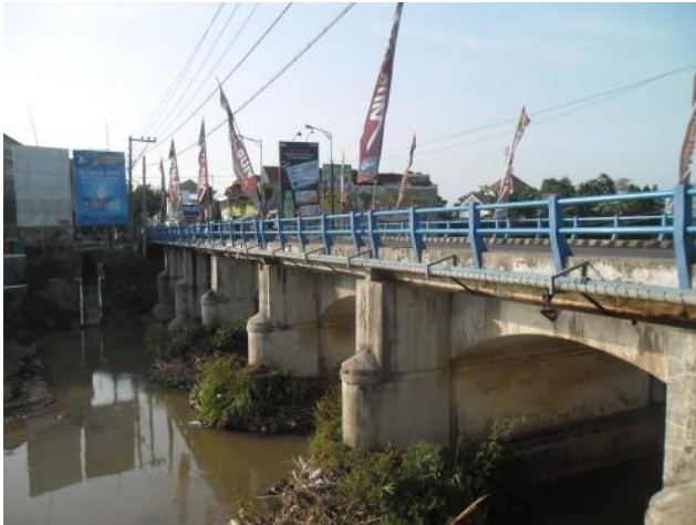
Picture 8. Condition of bridge of gelis river
