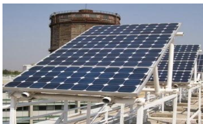
Gambar A.4. Panel Surya
