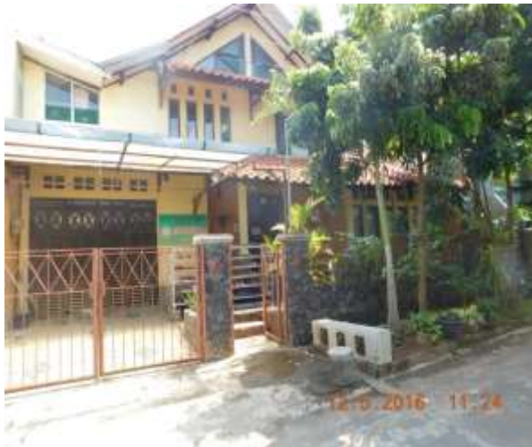
Picture of the dormitory of A7
