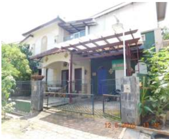
Picture of the dormitory of B5
