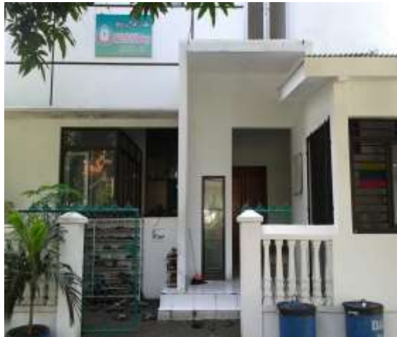
Picture of the dormitory of B9
