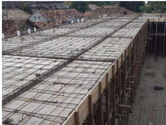
Gambar 4.20 atap dak beton (sumber : <https://indosarana.co.id/harga-borongan-dak-beton-per-meter/>)
