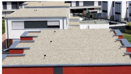
Gambar 4. 31 Contoh Atap Dak Beton
