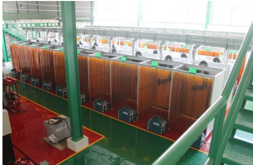
Gambar 4.11 Gedung bengkel pengelasan ( welding shop )
