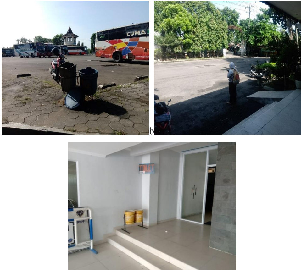
Gambar 3.3 Fasilitas terminal bus Purwodadi Grobogan
