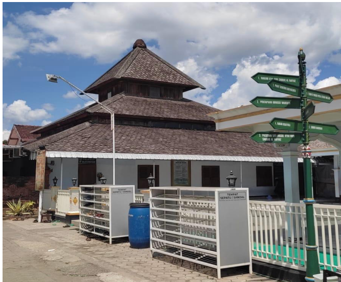
Image 3. 4 The roof of Tegalsari Jami Mosque.
