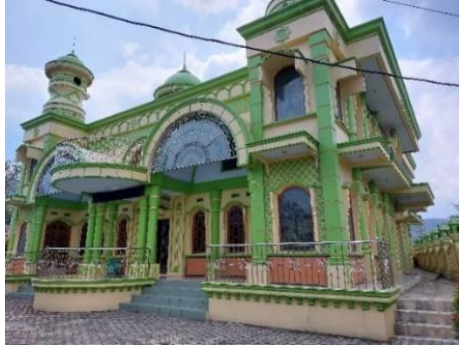
Masjid Arrohmah Walangsa
