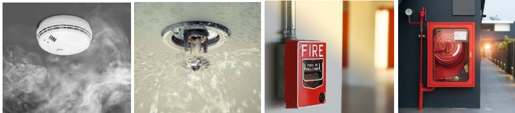
Gambar 4. 18 Contoh Smoke Detector, Sprinkler, Fire Alarm, dan Box Hydrant
