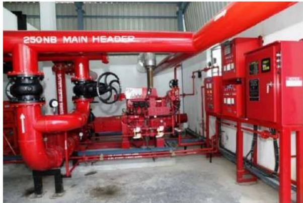
Gambar 68. Fire Hydrant System. Sumber: [depotsafety.co.id](http://depotsafety.co.id)
