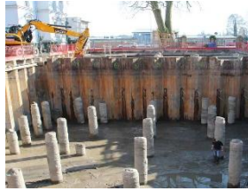
Figure IV-9 Pondasi Borepile (Sumber WEB Google)
